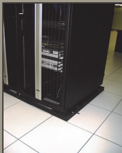
Platform under cabinet
