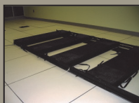
Platform before cabinet installation
