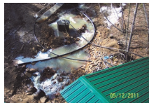
Zortman—DEQ Reclamation Equipment Flood Damage
